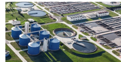
Biological Wastewater Treatment
